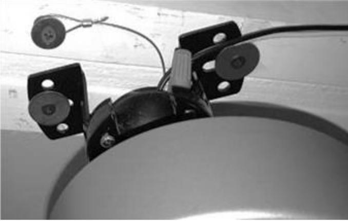
**Photo 8:** Safety cable attached near hanger
